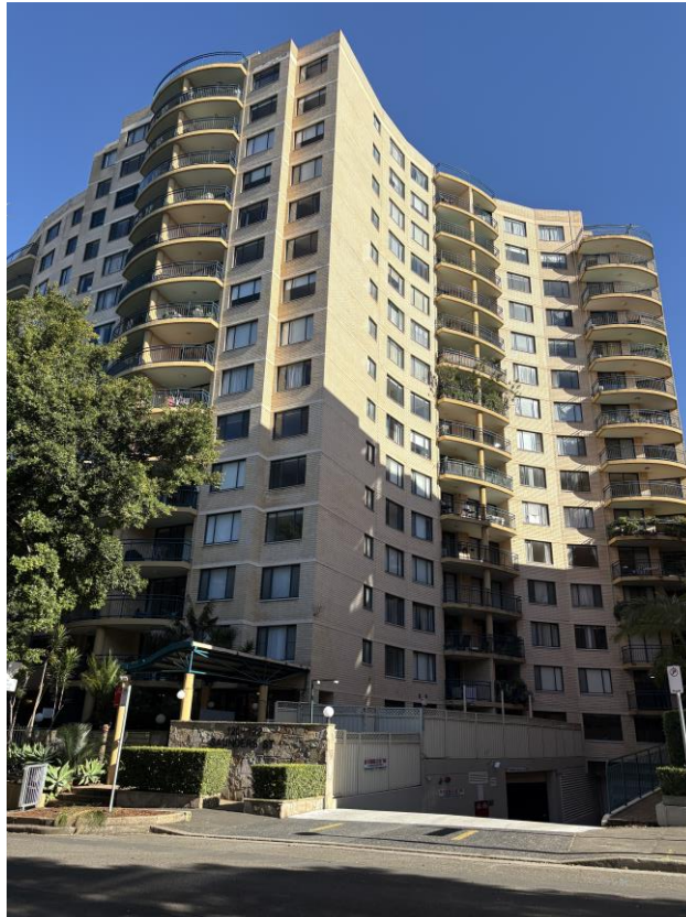
Figure 1: 120-122 Saunders Street, Pyrmont
